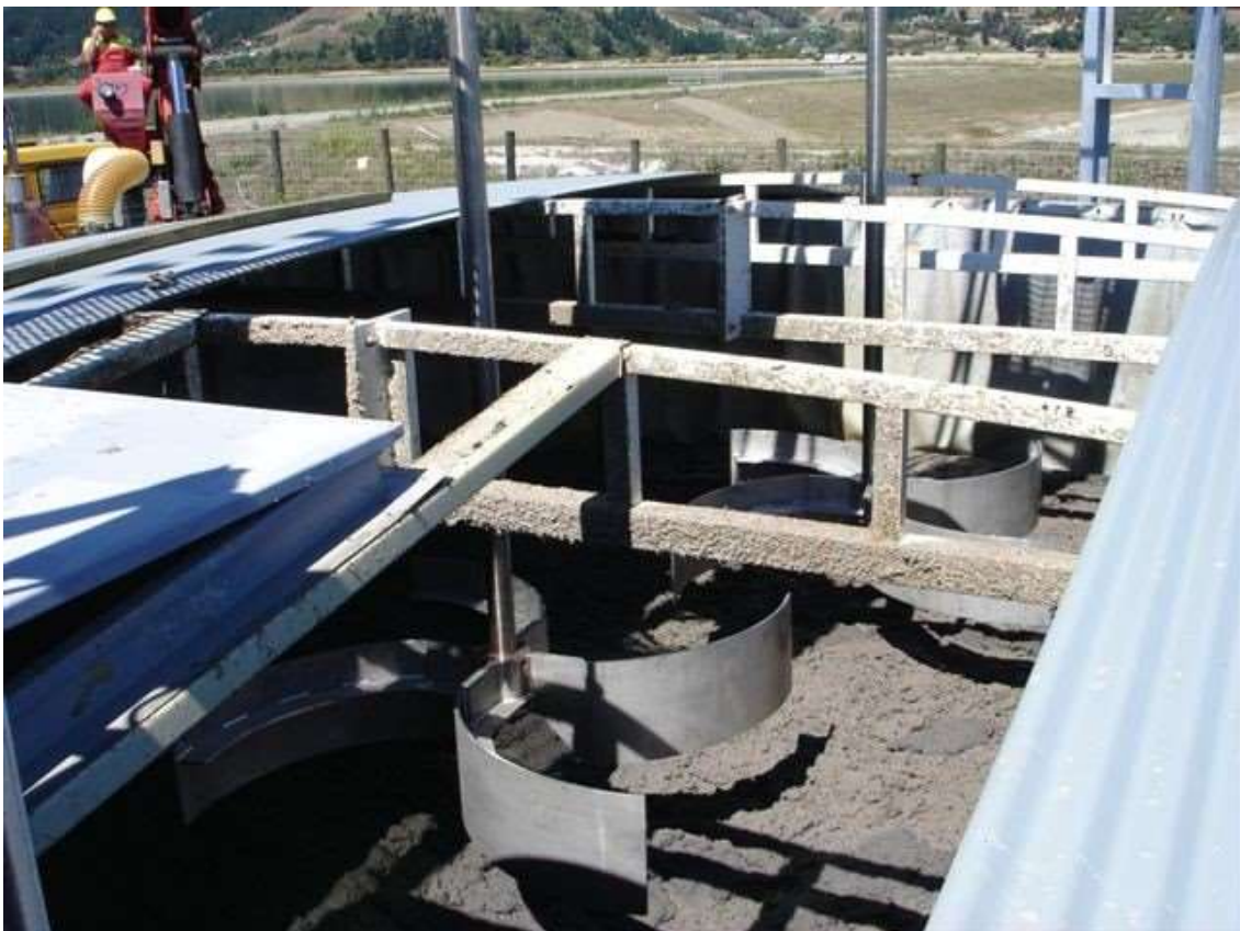
Mixtec Sludge Mixers in a Wastewater Treatment Plant
