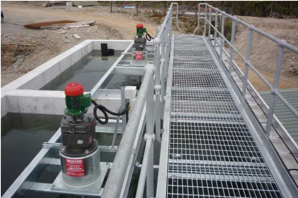
Mixtec Flocculation Mixers at Westport Water Treatment Plant
